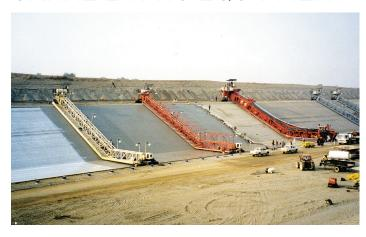
Guntert & Zimmerman pioneered the use of mechanized and automated canal construction machinery starting in 1947. Through the years, G&Z's canal equipment has proven itself to be highly durable and reliable. In regions of the world that rely heavily on irrigation such as the western United States, Spain and South Africa, G&Z equipment has been used to construct more than 80% of the existing concrete lined canals.
